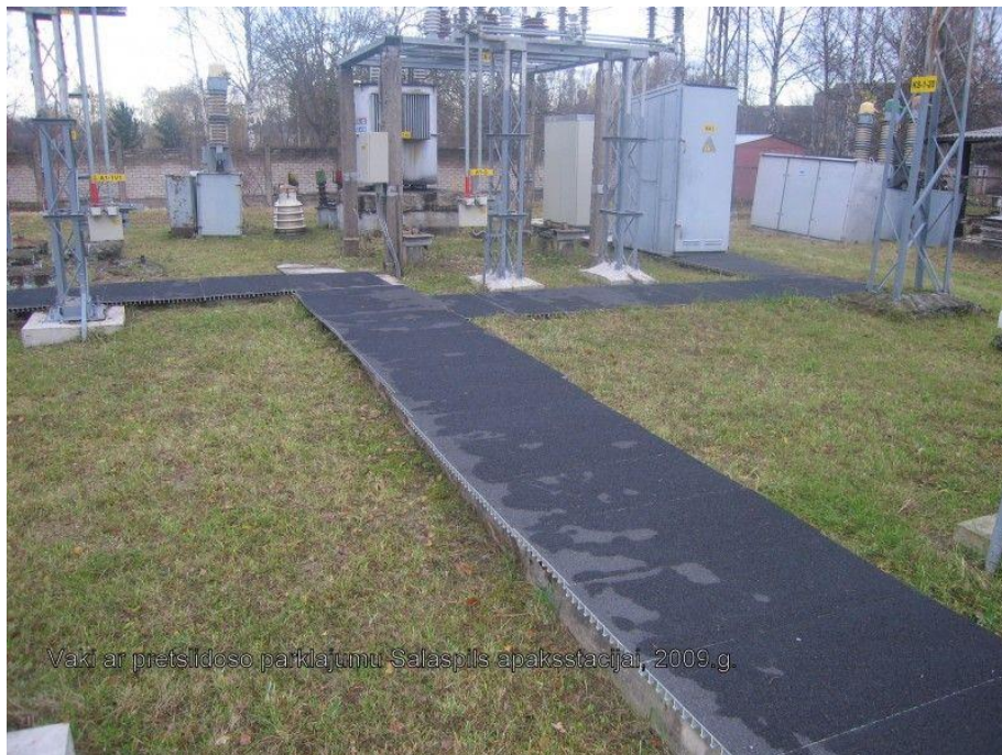
Fiberglass composite covers after renovation
