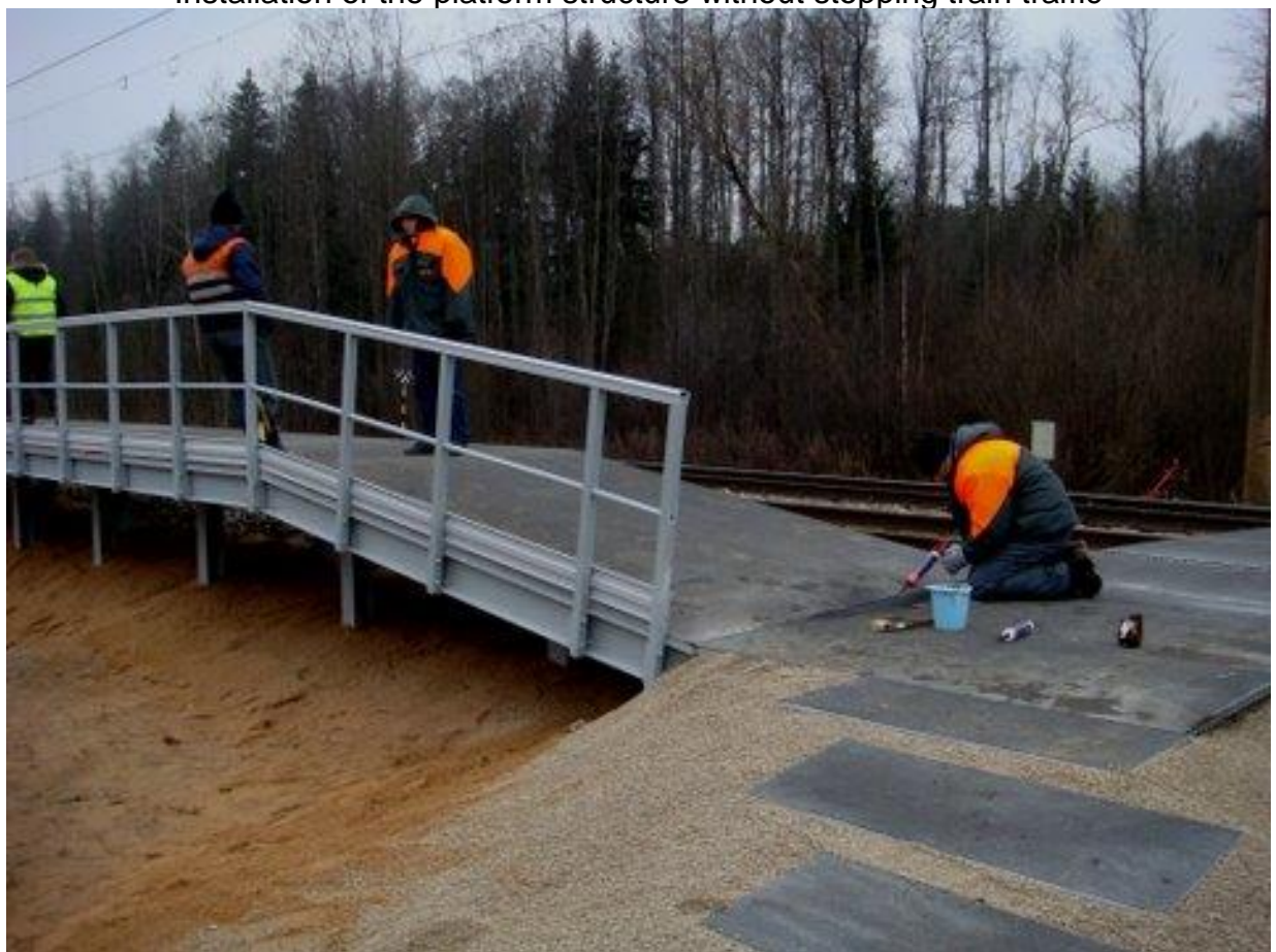
Installation of the platform structure without stopping train traffic
