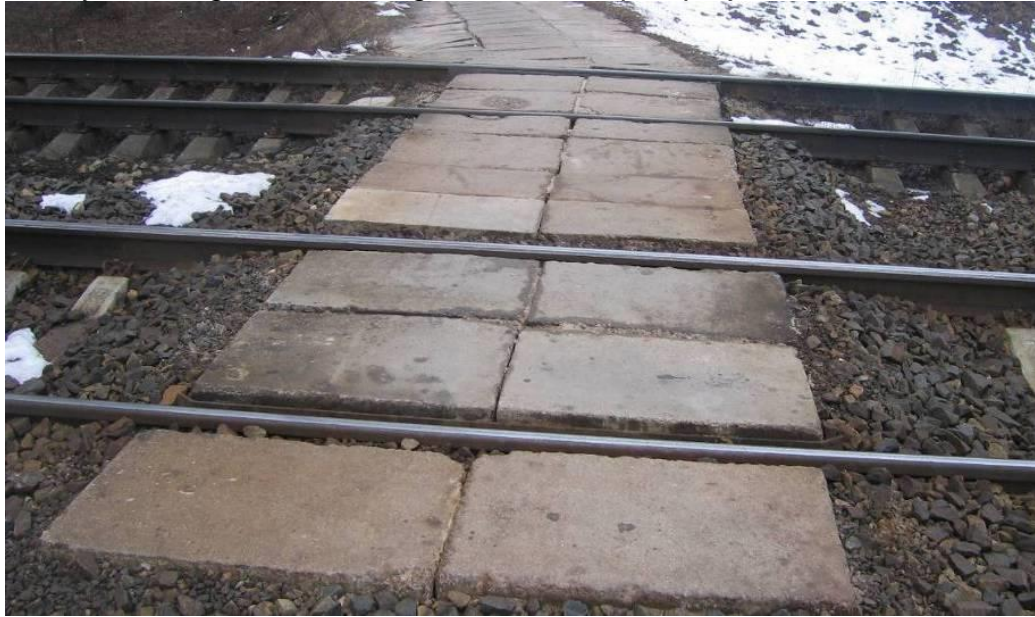
Railroad crossing made of concrete before reconstruction
