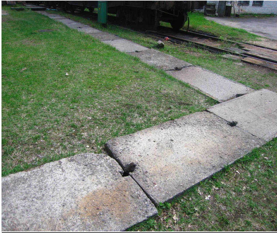
Concrete covers before reconstruction
