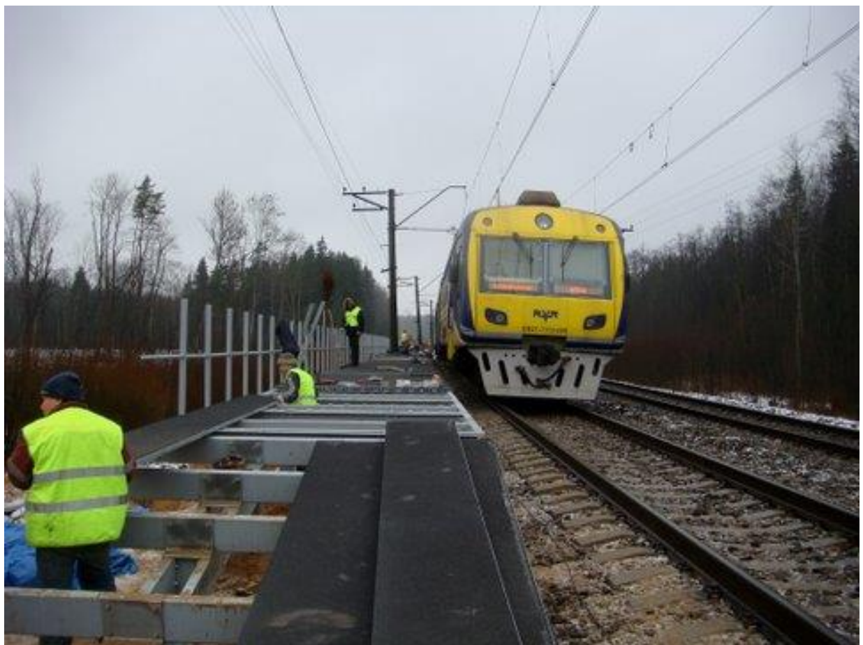
Installation of the platform structure without stopping train traffic
