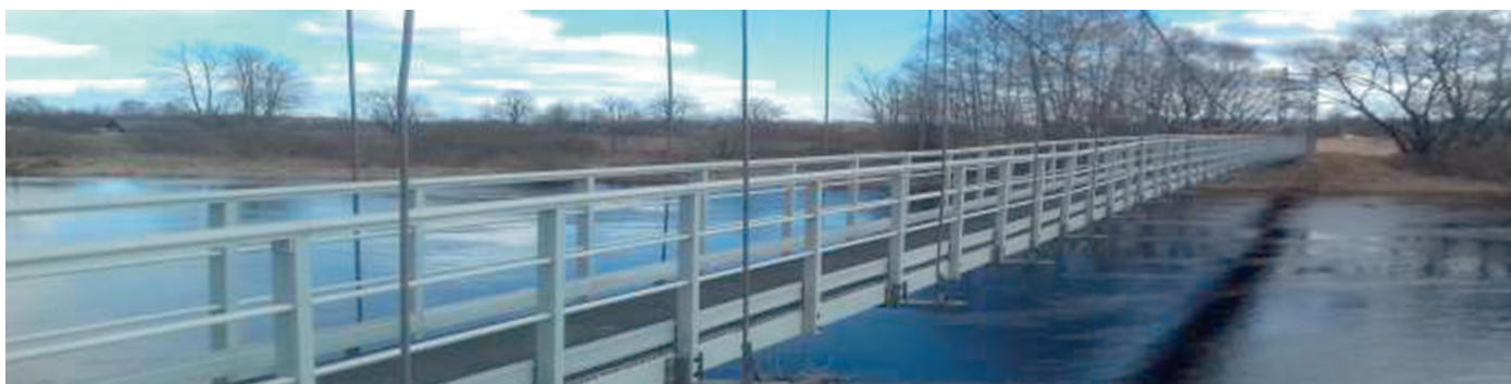
Bridge with concrete supports, joints and metal structures Pedestrian section and fencing made of fiberglass composite.
