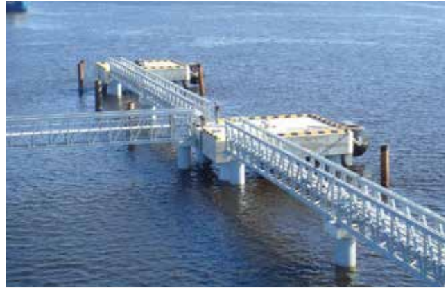
Ship service bridge, each section of 24 m
